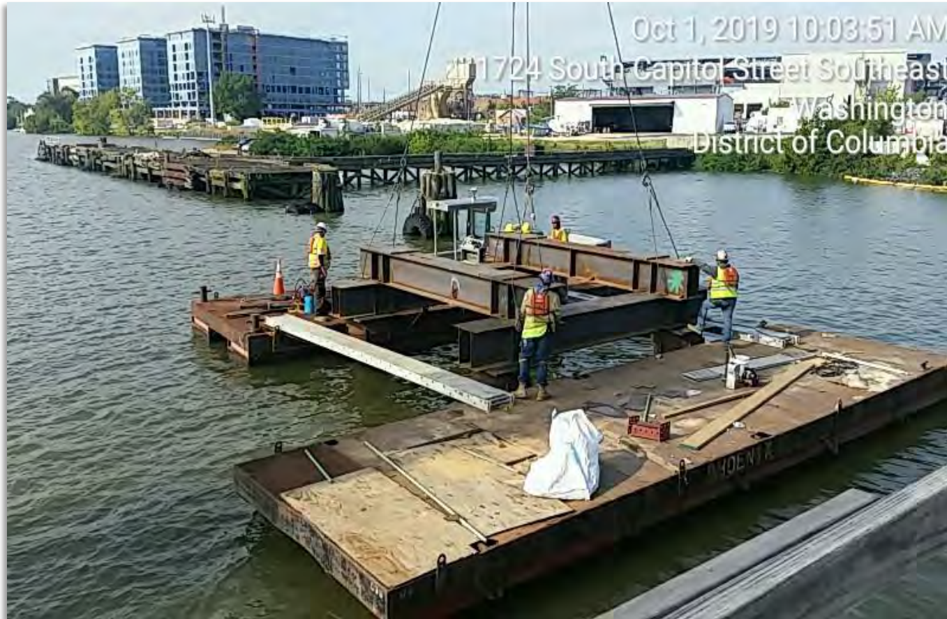
Arch span temporary support
