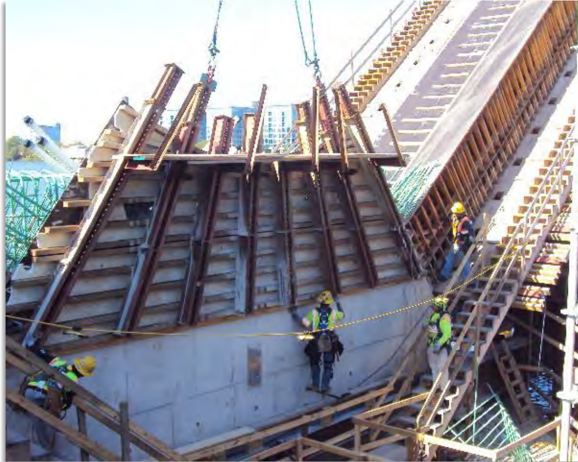
V - Pier 2 – Form Work and Reinforcing Steel Installation
